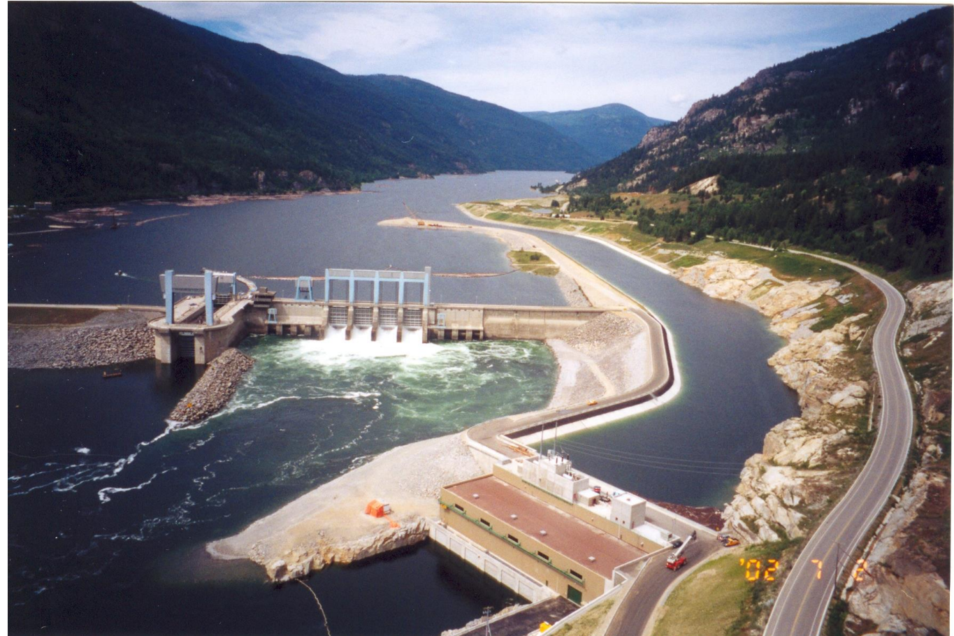
Hugh Keenleyside Dam near Castlegar
